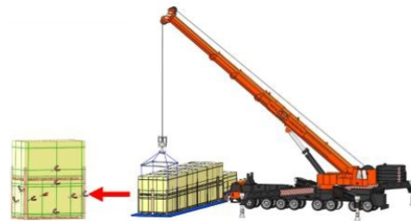
Vertical landscape package unloading with crane
